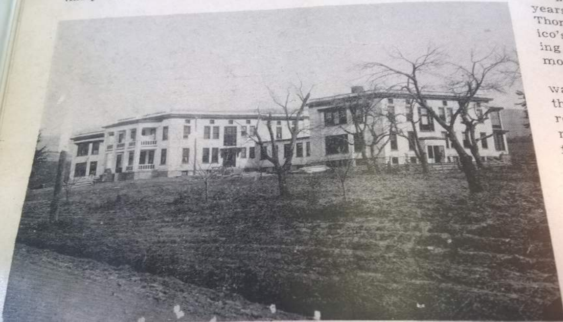
The New County Home Buildings
