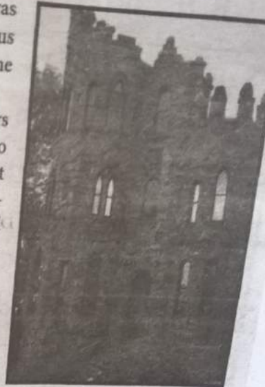
Built with stones from around the world. The Steinheim castle is one of the oldest buildings on the Alfred Uni- versity campus.
