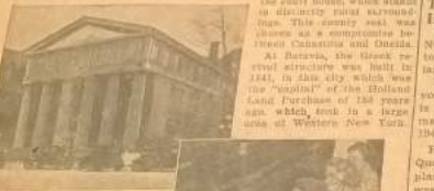
This classic structure of Cayuga County Court House at Auburn, N. Y., built in 1841, contrasts with much larger modern edifices of stone, the Queens County Court House, Jamaica, L. I., shown below.
