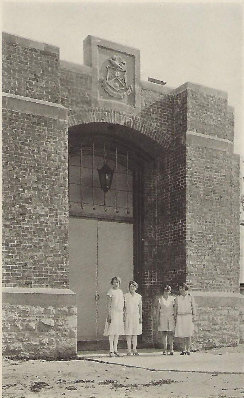
RECREATION BUILDING—MAIN ENTRANCE (NEARING COMPLETION JUNE, 1929)
