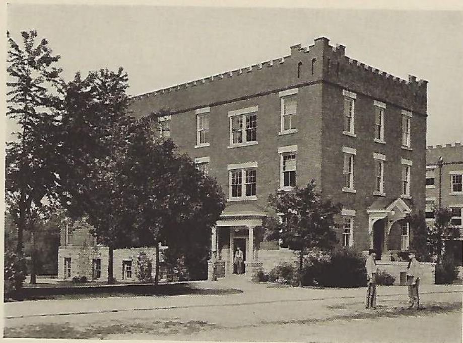
BARRACKS "D" (FIREPROOF) QUARTERS OF TWO INSTRUCTORS AND SIXTY CADETS
