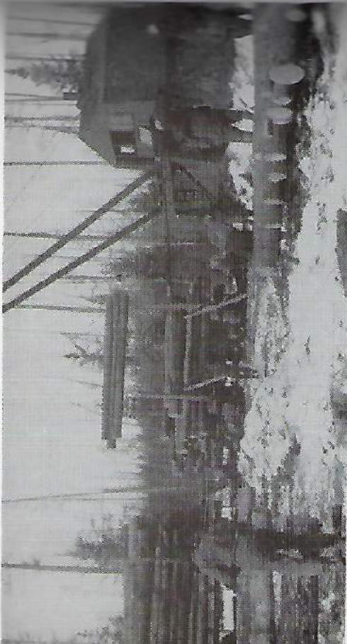
Courtesy Franklin A. King Loading cars with a Jammer at Camp 17 (Colbrath) on the Minnesota & North Wis. R. R. Note ralls over trucks of jammer over which empty logging cars were run through the jammer.
