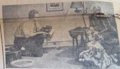
Record number of phones installed. The year's increase was 415,000, a new high. Although new applications for telephone service kept pouring in, we were able to reduce the waiting list from 436,000 to 276,000 during the year.
