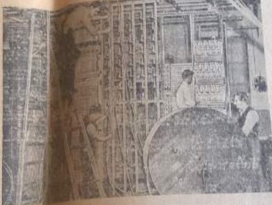
$155,000,000 was spent to expand and improve service. This is almost double the amount spent in 1946, and far more than in any previous year. Our construction program for 1948 calls for expenditures of about $170,000,000. (This photograph shows a small part of one of the 40 new central offices added during 1947.)
