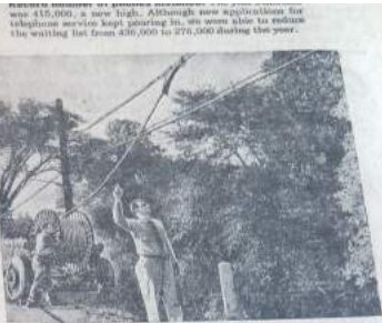
Construction program the biggest in our history. Our manufacturing and supply unit, the Western Electric Company, turned out switchboards, cables and other complicated apparatus in tremendous volume. 1,500,000 miles of wire in new cables were placed in service so that more telephones could be connected.
